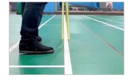
Peel the masking tape after paint dry.
