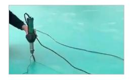
Welded seams must cool to room temperature before trimming in two steps, rough and fine trimming.
