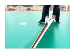
Remove the release film on the other side of the tape and stick two pieces of flooring onto the tape.
